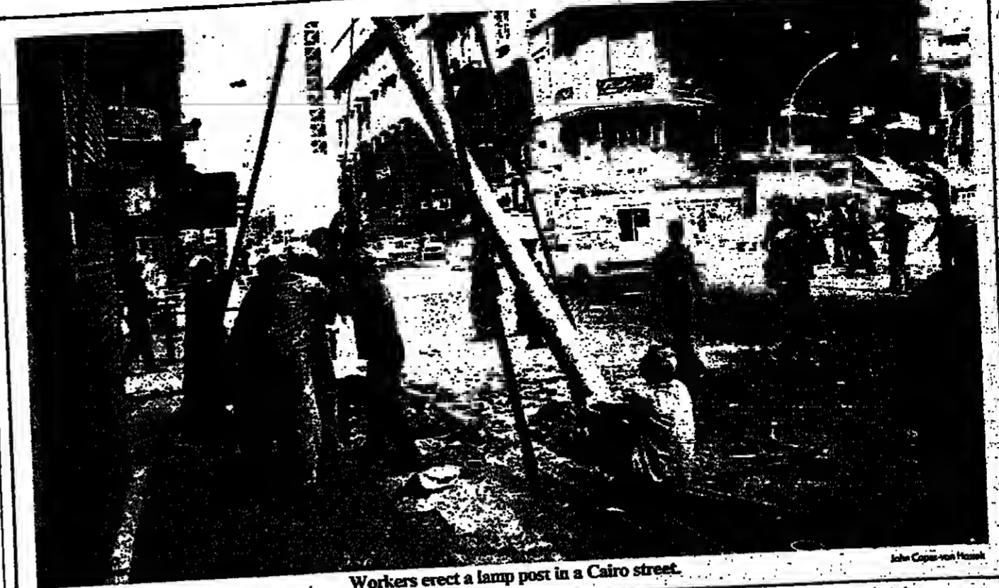
Workers erect a lamp post in a Cairo street.
